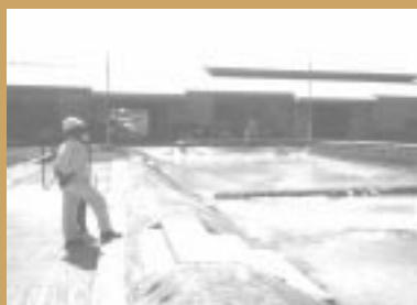
Wastewater treatment facility of a locator company in PNOC, Bataan
